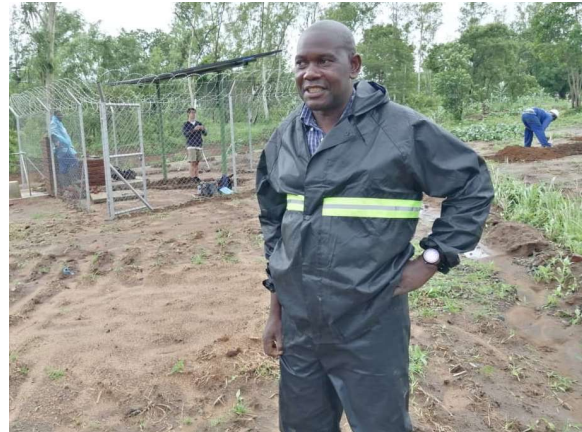
Brother Goodson supervises work on site
